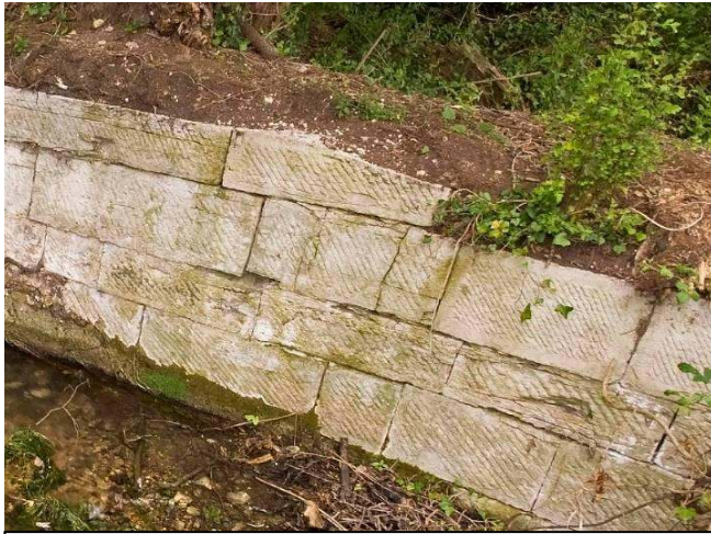
Dressed stone with tooling on vertical faces (Photo © Dennis Bright)
