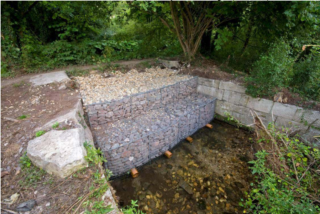
After installation of the stone-filled gabions by Dennis Bright (Jul 2010)
