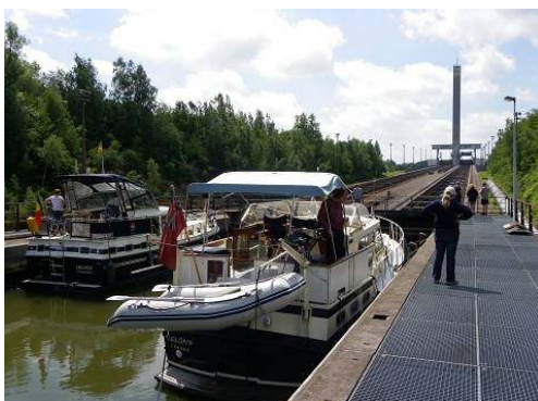
Elsa in the tank rising up in the Ronquières Ship Lift
