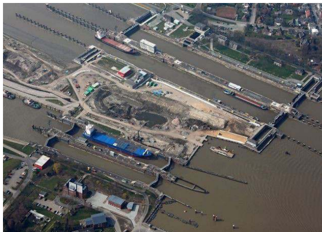
Brunsbüttel lock complex with new lock construction (Photo-WSA-Brunsbüttel)
