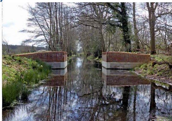
The new section of canal available for restoration is south of this new bridge at Birtley, where in the next few months volunteers will be adding the deck.
