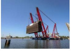
the heavy lift vessel Gulliver of Jan De Nul Group can now lift the door out of its position. The 'Gulliver' is a pontoon derrick that can lift a weight of over 3,300 tonnes. The whole operation is a sequence of several partial operations that have been meticulously planned and prepared. The works started at 3 o' clock at night and will take an estimated 19 hours.
