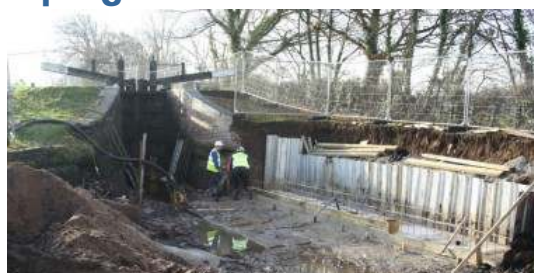
Winter works at Quoisley Lock on the Llangollen
