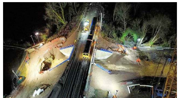
Below: The track has been relaid - 31 December 2021
