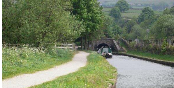
Western entrance to Standedge Tunnel
