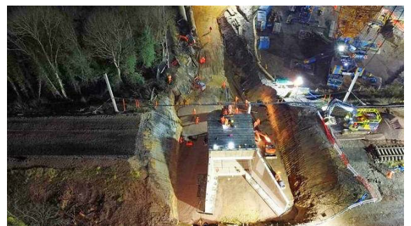
Above: The new culvert in position - 29 December 2021
