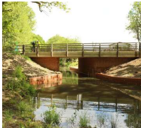
Right: The new bridge
