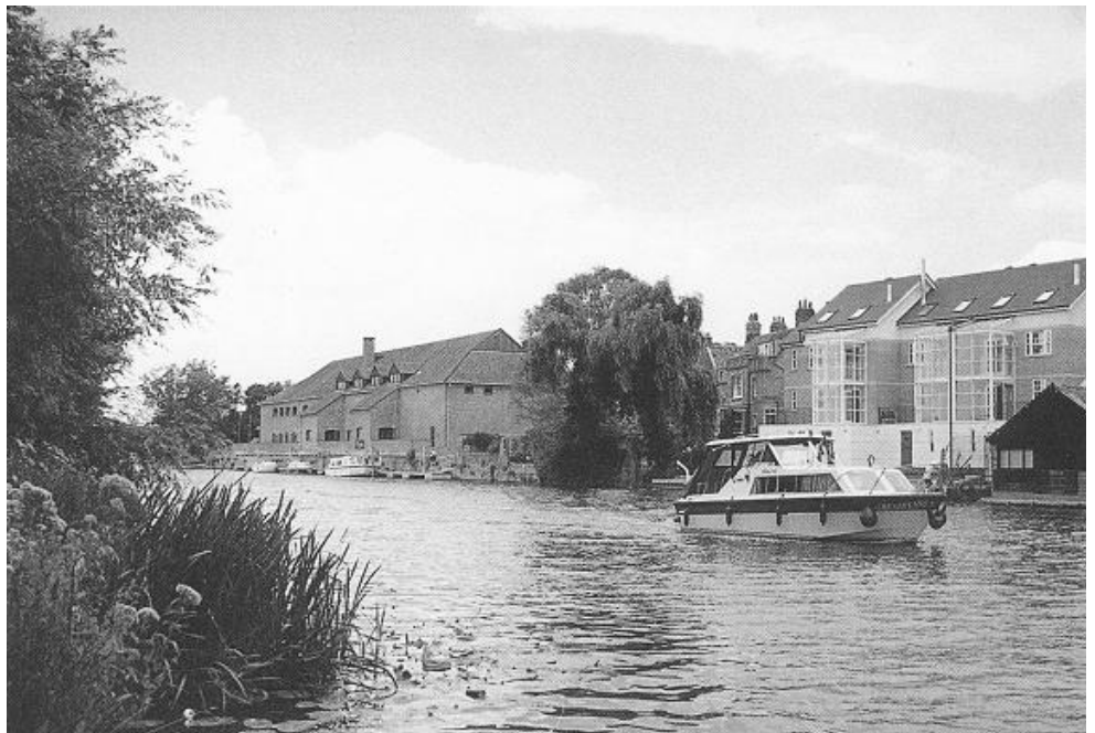
The Swan House, Priory Terrace, St Neots is Hugh's new house overlooking the River Great Ouse (the one on the right, with a conservatory over 2 floors)
