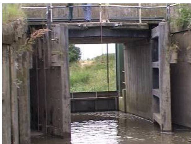
Above: An outer set of mitred gates or doors exists on the other side of the bridge at Old Bedford Sluice to keep out high tides on the Great Ouse.
