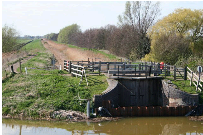
Above: Welches Dam Lock in 2007 with the Forty Foot Drain stretching away in the distance and is now an unnavigable reed bed.
