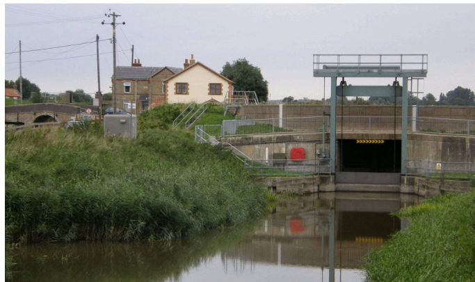
Below: The inner guillotine gate at Old Bedford Sluice in 2007. This gate replaced a pair of mitred gates in 1996. On the left of the picture is the bridge over Salter's Lode Lock on Well Creek.
