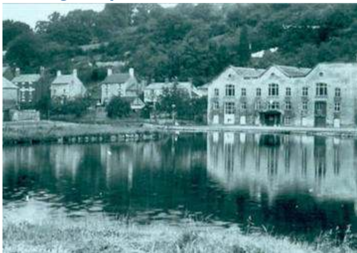
Above: Brimscombe Port before infilling (photo: Stroud District Council) Below: Brimscombe Port CAD (computer-aided design) drawing of new port seen in the same general direction as above but from a different elevation.
