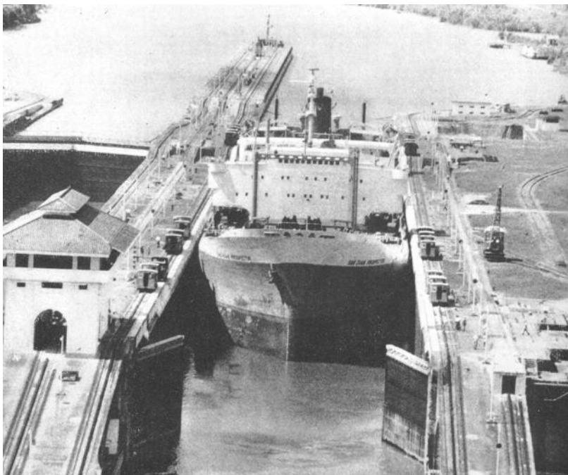
A ship squeezes through one of the 110 ft wide locks on the Panama Canal
