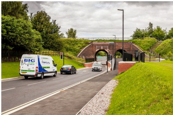
Above: James Street Aqueduct after repairs (Photo: Mark Edwards)
